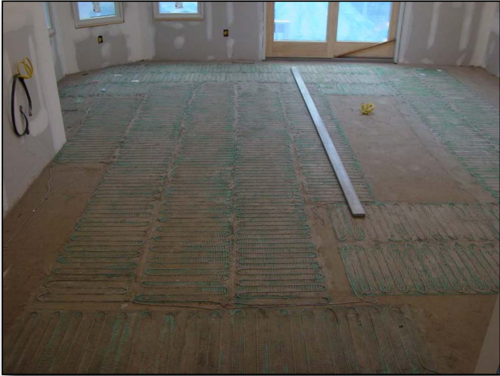
Electric radiant heat and porcelain floor install.
